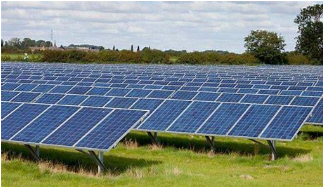
Figure 11: Single access tracking solar farm with bi-facial panels 7
