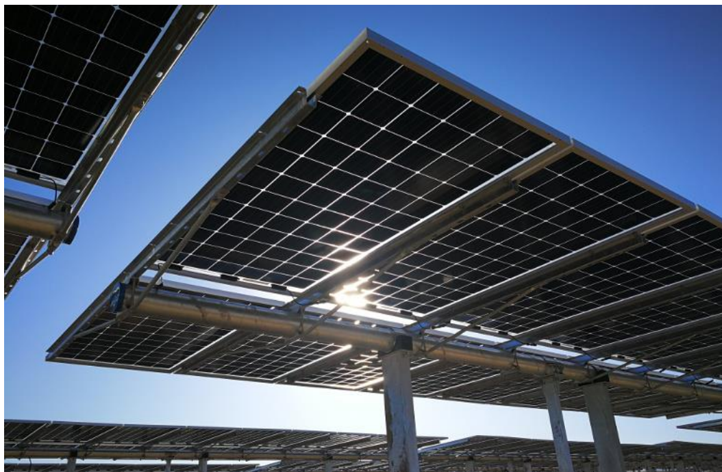
Figure 11: Single access tracking solar farm with bi-facial panels 7
